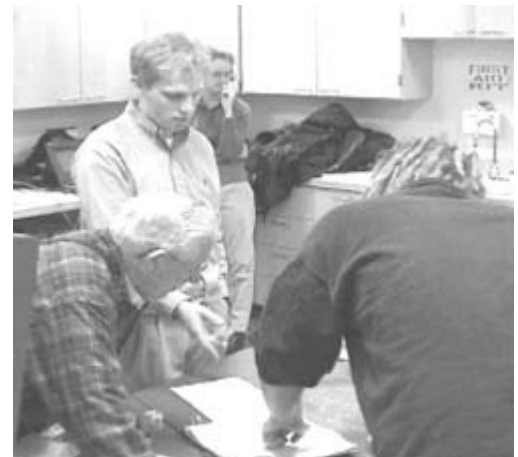
Bud Hardman, Nate Dudley, and Collin review mechanical plans while construction goes on around them in the machine shop.
